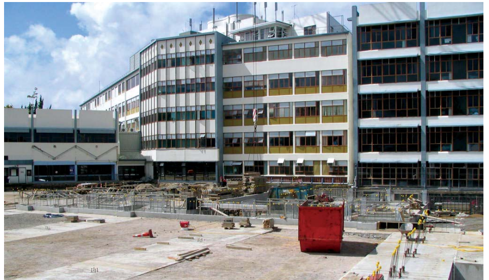
Tauranga Hospital under construction
